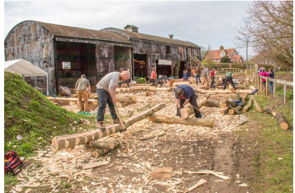
Volunteers and members of the Carpenter's Fellowship working on the timber frame for the House of Wessex
